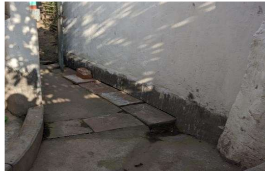
(Fig. 7 & 8. open and covered drainage system in the Kareya village, Purulia)
